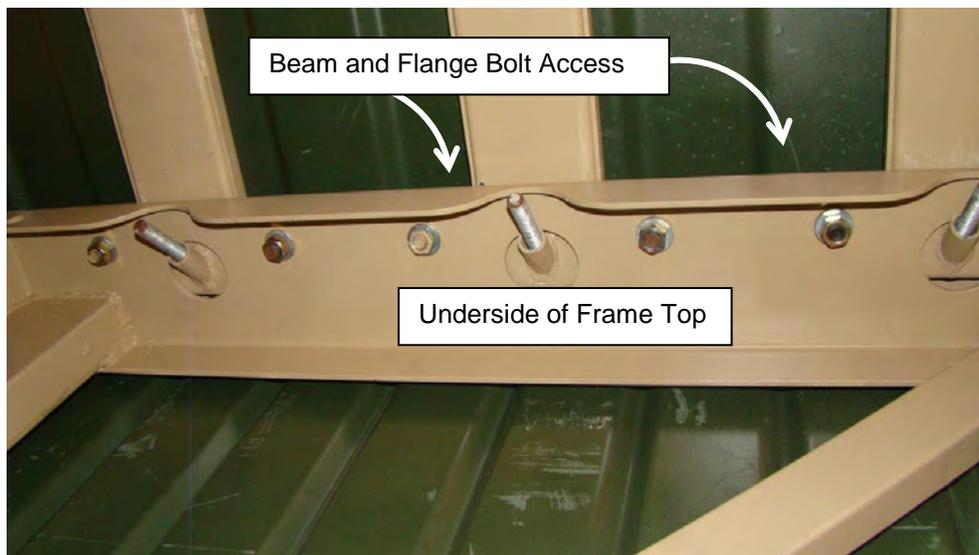
15. With the frames and beams in place, tighten (with a  $\frac{3}{4}$ " open end wrench) all the top and bottom bolts and nuts on both sides of the frame works.
