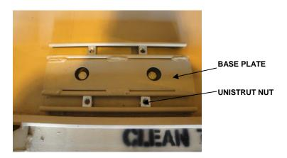
13. Remove unistrut channel nuts from mounting channels in ceiling.
