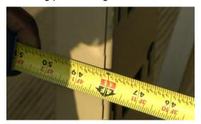
8. Install the *third* vertical rack following steps 3 through 5 above. Measure **30-inch** from the inside of the second rack to the inside of the third rack. Once the correct measurement is verified at all four points on the vertical rack frame, tighten the bolts on the top and bottom mounting plates using a ¾-inch socket and ratchet.
