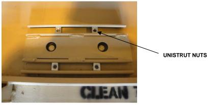
22. Remove unistrut channel nuts from mounting channels in ceiling.
