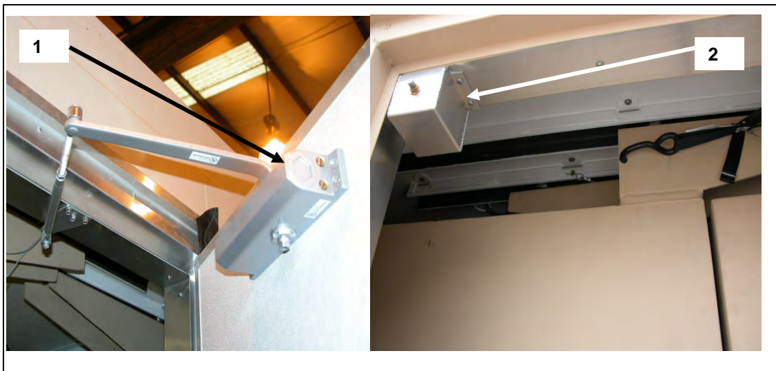
Figure 4.3-1 Door Damper and Door Light Switch
