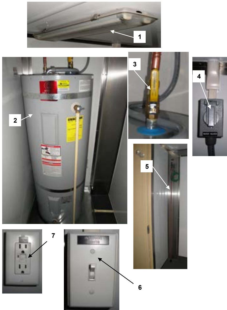
FIGURE 06 CONTAINERIZED SHOWER UTILITY ROOM COMPONENTS
