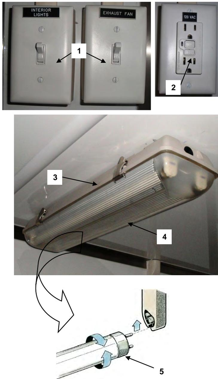
FIGURE 05 CONTAINERIZED SHOWER INTERIOR 6 COMPARTMENT ELECTRICAL
