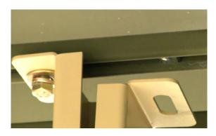
6. Install vertical rack frames from right to left beginning with the *first* vertical rack at the far right. Measure **8 1/8-inch** from the inside of the container frame to the outside of first vertical rack frame. Once the correct measurement is verified at all four points on the vertical rack frame, tighten the bolts on the top and bottom mounting plates using a ¾-inch socket and ratchet.
