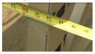
9. Install the *fourth* vertical rack following steps 3 through 5 above. Measure **48-inch** from the inside of the third rack to the inside of the fourth rack. Once the correct measurement is verified at all four points on the vertical rack frame, tighten the bolts on the top and bottom mounting plates using a ¾-inch socket and ratchet.
