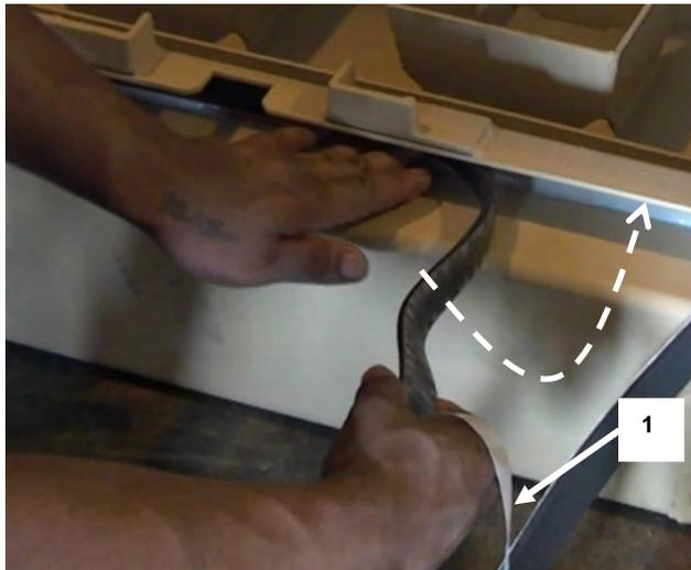
5. Peel back the paper backing (1) as you place the seal in position.
