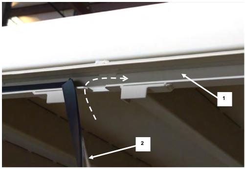
**NOTE** Seals should not be stretched, but positioned in a relaxed state.
