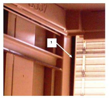
1. The left side and right side inner frame seals (1) are applied to the inner edges (2) in the same fashion as the upper frame seal and trimmed at the end of the run (3).
