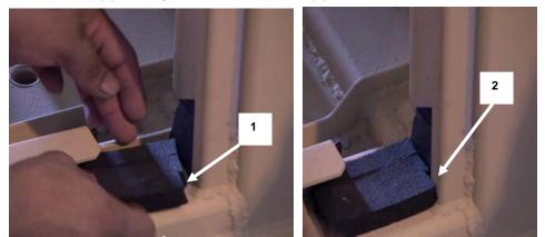
5. Cut a notch (1) and dry fit the bottom corner (2).
